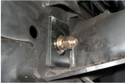
21. Picture shows inner frame bracket & hardware installed.
