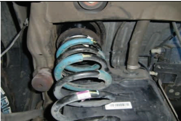
Reinstall isolators and coil springs and raise axle
