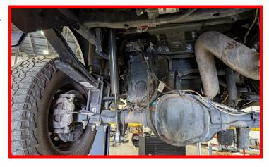
If equipped with a 2 piece driveline, remove the bolts holding the carrier bearing to the frame. Install the ReadyLIFT carrier bearing spacer between the carrier bearing and frame using 7/16" bolts, washers and a drop of thread locker. Torque to 50 ft-lbs.
