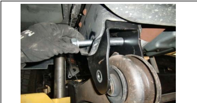
17. Stage 1: Install new radius arm drop brackets.
