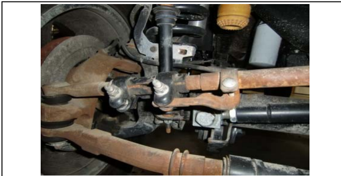
103. 5) Tighten up the hardware and replace the keeper bolt.
