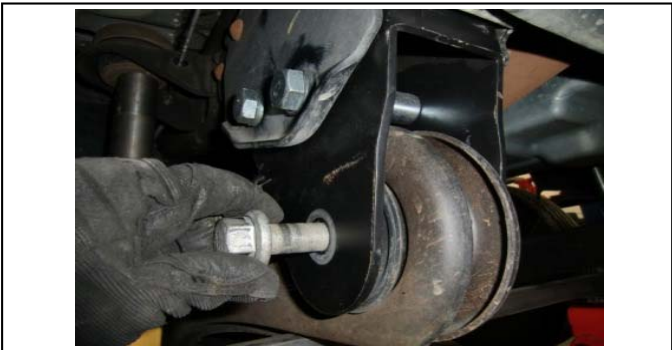
18. Stage 1: Raise the radius arms and reattach to the drop brackets.
