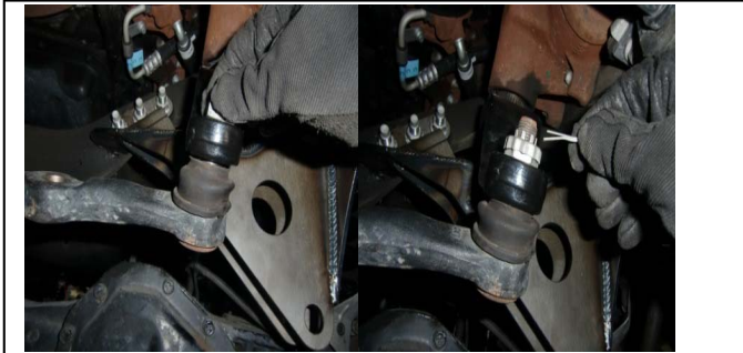
42. Install the drag link to the new drop pitman arm and torque. Replace the keeper cap and cotter pin.
