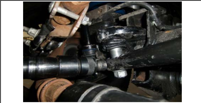
51. Use the ball joint fork/air hammer to separate bar from ball joint.
