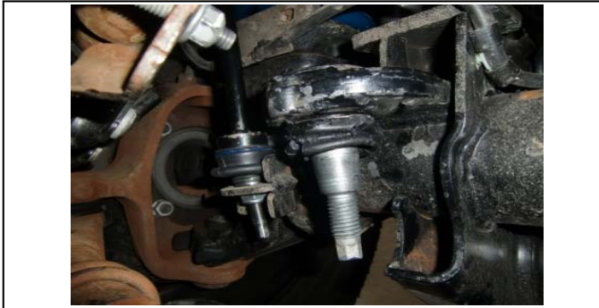
52. View of the ball joint to be removed.
