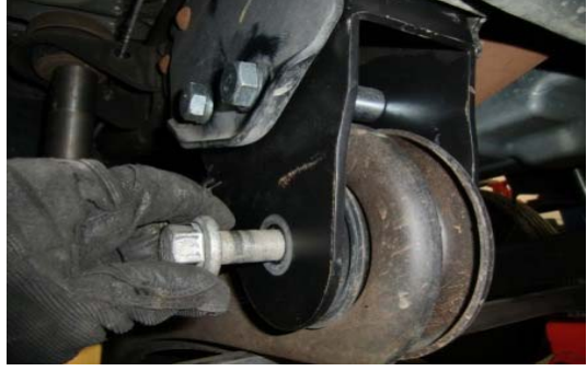
18. Stage 1: Raise the radius arms and reattach to the drop brackets.
