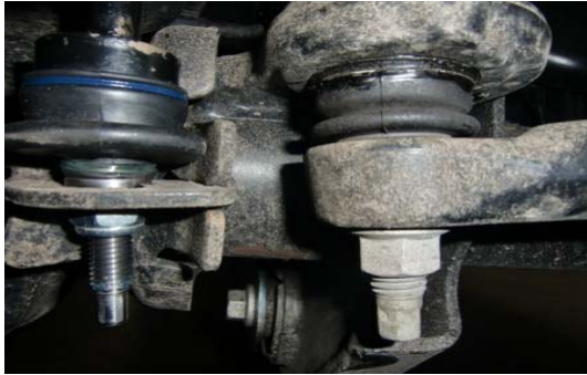
49. Stage 3: (Steps 49-69) View of track bar ball joint at axle mount.
