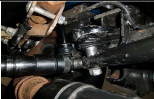
51. Use the ball joint fork/air hammer to separate bar from ball joint.
