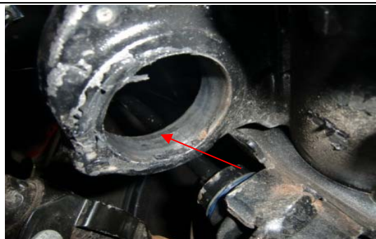
56. Inspect and clean the surface and edges.
