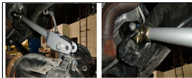
15. Install the new arm into frame and onto axle, then tighten down. You may need to un-bolt the passenger side to fit the Driver side arm due to length differences from stock arm to ReadyLIFT® arm.
