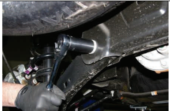
Remove inner lower control arm hardware.
