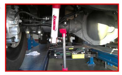
Loosen but do not remove the U-bolts on the passenger side. Remove the U-bolts completely from the driver side. Discard the factory U-bolts, washers, and nuts.
