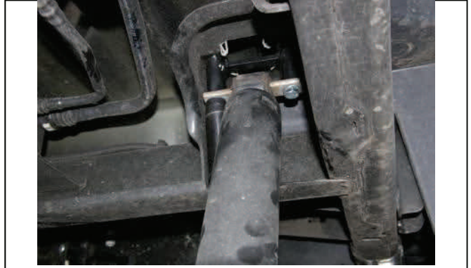
Install new upper shock extensions with new hardware
