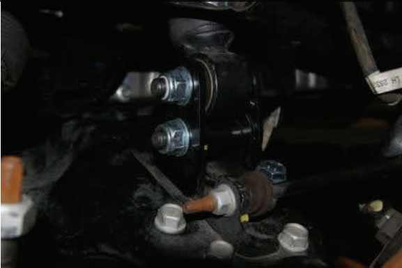
Reinstall strut with new hardware on bottom and OE on top
