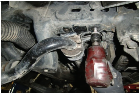
Disconnect sway bar at the frame mounts.
