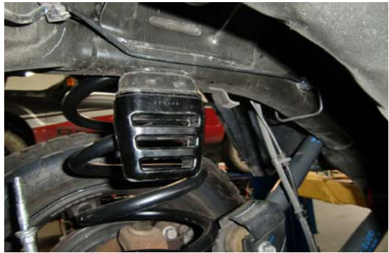
New bump stop installed correctly.
